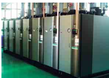
New natural gas-fired boiler (The Yamakita plant)
