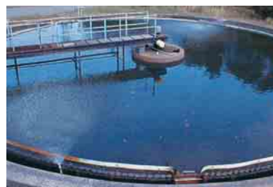
Settling tank in activated sludge system
